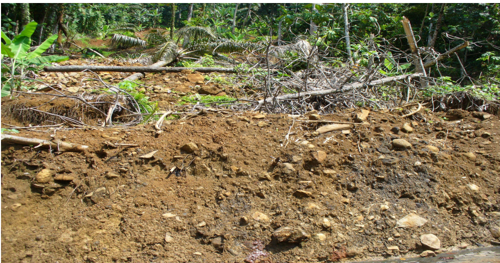
Image 2- Erosion, with landslides Angra Toldo Cavalete Caué
