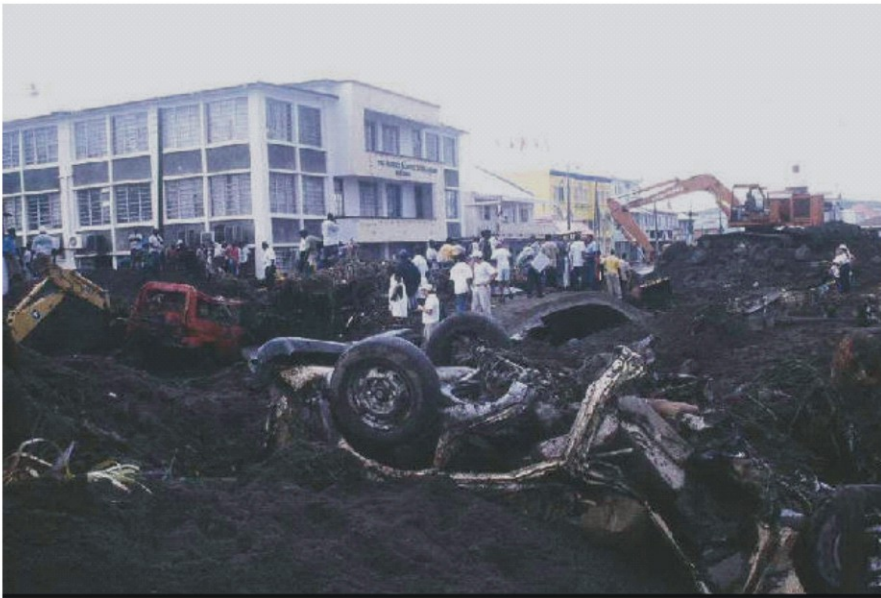
Figure 42: Aftermath of Flooding
