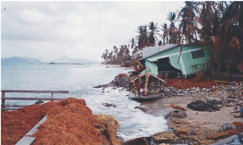
Figure 41: Major deposits of seagrass; damaged property and loss of sand due to a severe hurricane
