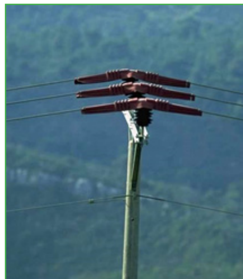
Plastic isolation put on the power-line pole. Photo: V.Radek
