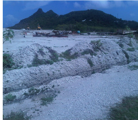
Construction of Marina in Carriacou June 2009
