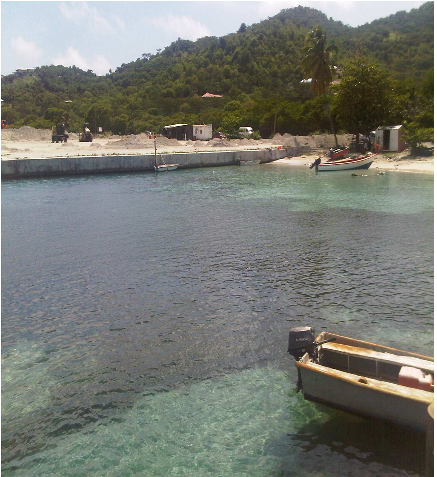
Jetty Construction in Grenada
