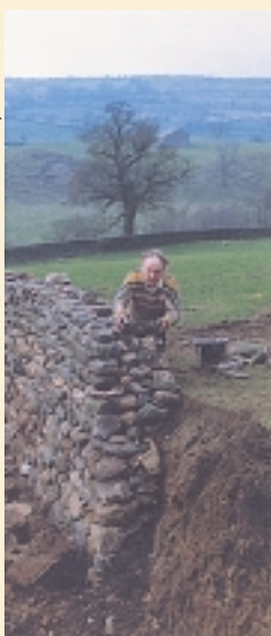
Dry stone walling, a traditional way of building field boundaries, contributes to the distinctive character of the Yorkshire Dales.
