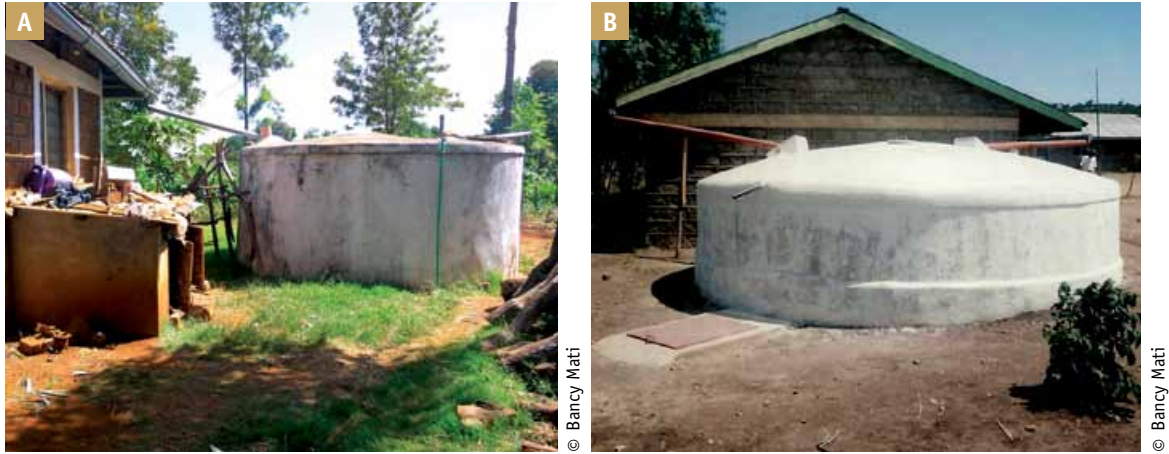
Photo 20. Structures for water harvesting: (A) Roof catchment tank for household water in Embu, Kenya; (B) Rainwater harvesting from roof catchment for institution in Nyando, Kenya
