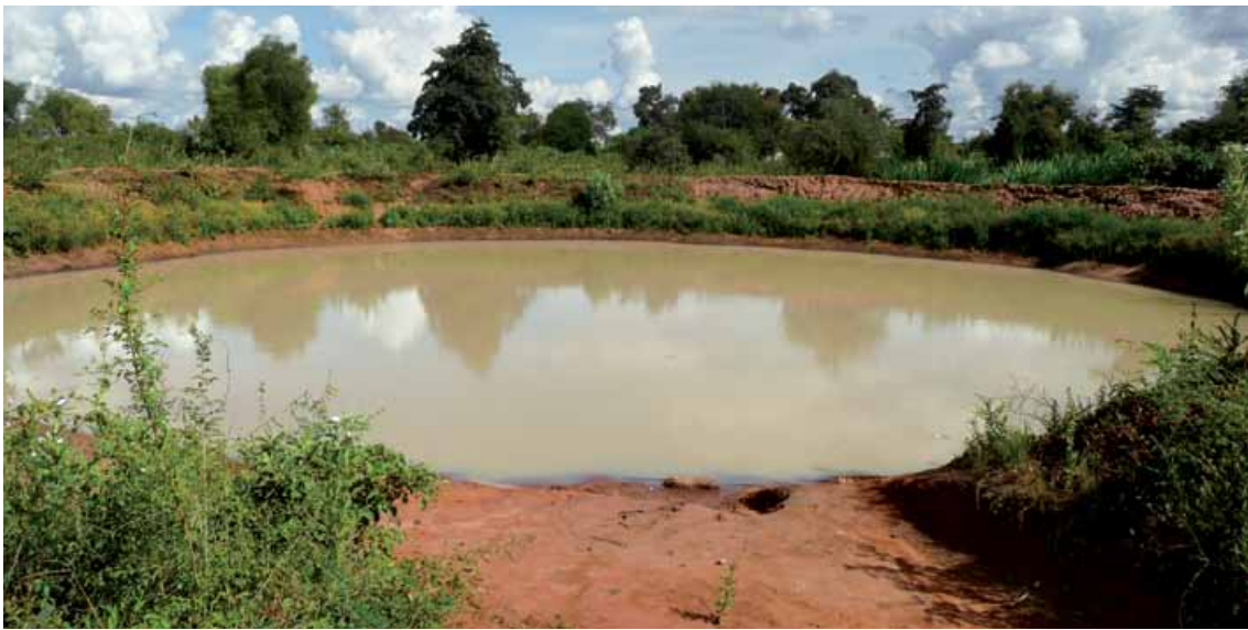
Photo 19. Road runoff harvesting into pan
