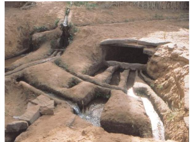
Oasis de Ouled Saïd Ramsar site 1060 Adrar; Algeria. A rare human-made wetland created on the vestiges of a "fossil" wadi consisting of a fougara , an ingenious system for the capture and distribution of groundwater.
