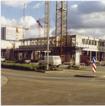
Setting up a Center... ZEF building in 1989
