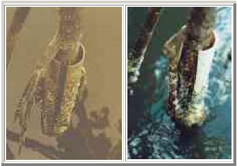
how the split will continue to enlarge. The first photo was taken in February 1995 and the other in February 1997. It is this progressive widening of the longitudinal split that facilitates the principle of spontaneous adaptation in REM methodology.
