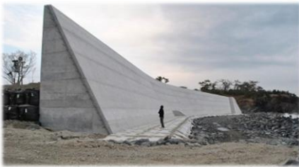
Gigantic coastal levee being built in tsunami-affected area
